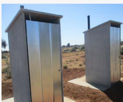
VIP TOILETS AT LORATO VEGETABLE FARMING CO-OP
