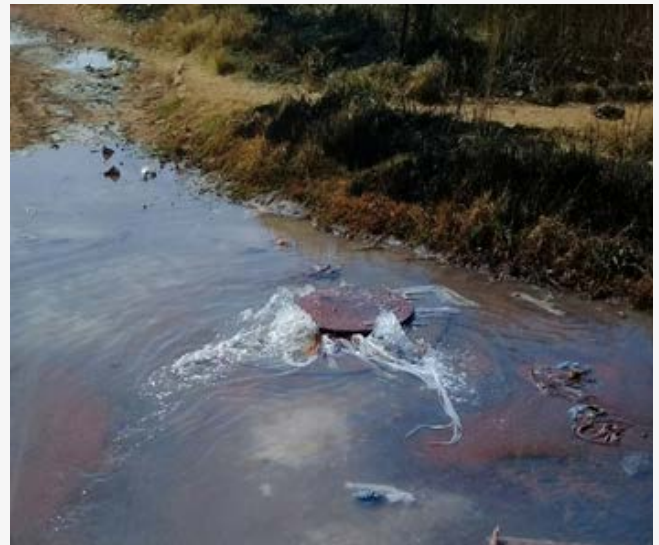
Sewer Spillage by Thamsanqa Primary School Orange farm Ward 1
